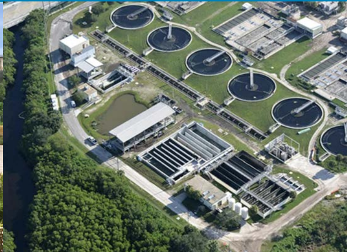
Megamix II with Bio-San: Largo Wastewater Treatment Plant - USA
