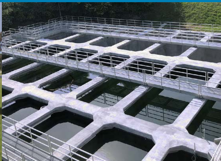
Megamix II: Mitchell Water Treatment Plant - USA
