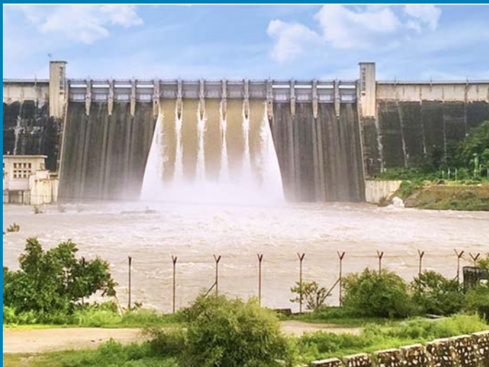
Patch'n Plug: The Rihand Dam - India
