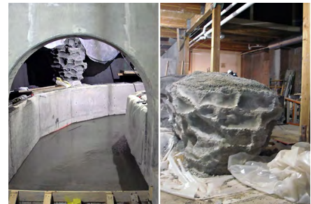
Fig 5 -- The Shark Gallery & SeaTube exhibit begin to take shape. Every tank and feature in the aquarium used concrete treated with Xypex Admix C-500 to provide waterproofing and chemical protection.
