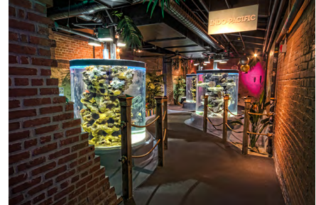
Fig 6 -- Concrete bases and walls were treated with Xypex Admix C-500 to provide integrated and maintenance-free waterproofing for the life of the aquarium. The circular concrete aquarium bases in the Asia & Indonesia exhibit received custom-made acrylic tanks (see inset photo).
