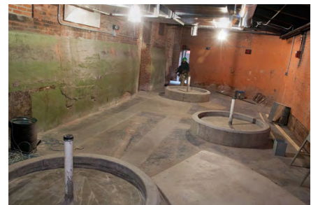
Fig 5 -- The Shark Gallery & SeaTube exhibit begin to take shape. Every tank and feature in the aquarium used concrete treated with Xypex Admix C-500 to provide waterproofing and chemical protection.
