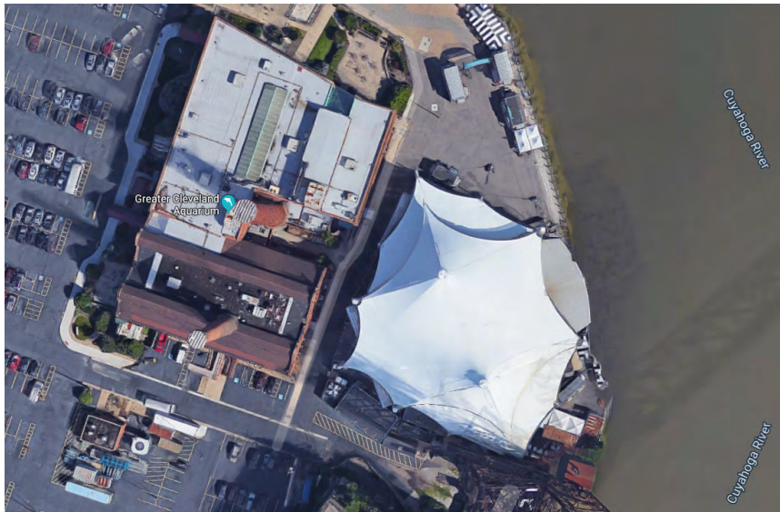
Fig 4 -- Located in the Flats area along the west bank of the Cuyahoga River, the Nautica Entertainment Complex is home to multiple restaurants, the Jacobs Pavilion (tent structure) and the Greater Cleveland Aquarium.
