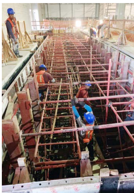
Preparation of Cistern
