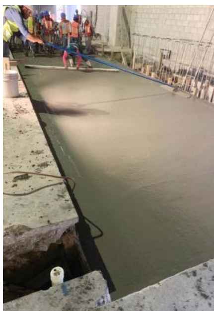
Finishing of Cistern slab
