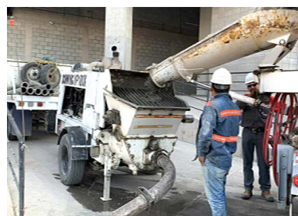
Pouring Xypex Admix treated concrete
