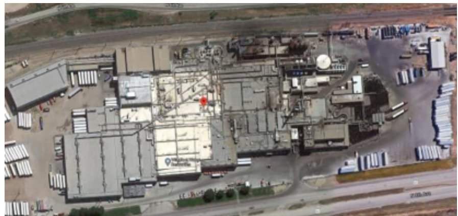
Fig 2 -- JBS USA Greeley, Colorado beef processing plant encompasses more than 850,000 ft 2 of production space.
