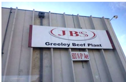
Fig 1 -- The JBS USA beef processing plant has more than 850,000 ft 2 of production space. Most of the plant is constructed of tilt-up precast concrete walls on concrete slab floors.
