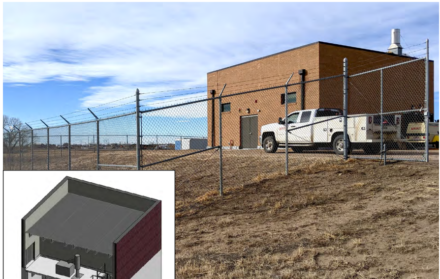
Fig 4 -- The Lamar, Colorado, headworks facility was built in 2010 to replace a lift station that had reached its end of life. Within a few years, the facility experienced significant corrosion due to excessive level hydrogen sulfide produced by the slow moving waste stream. In less than 10 years, a major restoration was required. Inset: Two-thirds of the Lamar headworks facility is located below grade, resulting in constant hydrostatic pressure from ground water.
