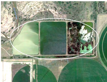
Fig 3 – The Lamar headworks facility is located about 1.5 miles (2.4 km) west of a three-cell lagoon system (circled). Wastewater is pumped from the headworks to the lagoons via a 24 inch (.6 m) force main pipeline.
